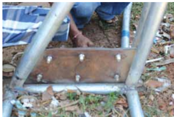
Fig.7. Assembling the 12 m cage in the beach
