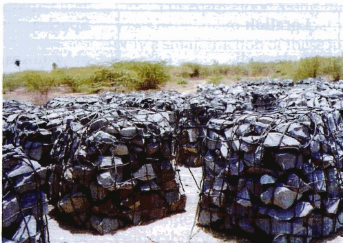
Gabion Box filled with stones
