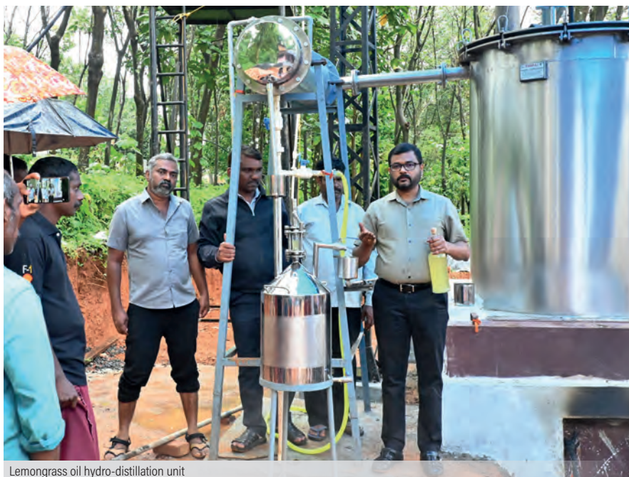
Lemongrass oil hydro-distillation unit
