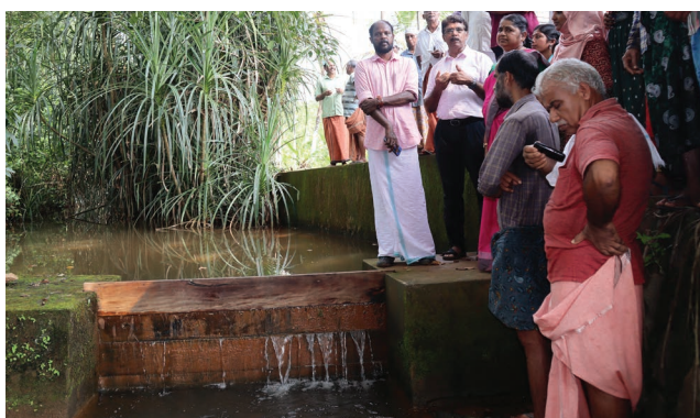
Wooden plank installation at Chuzhali
