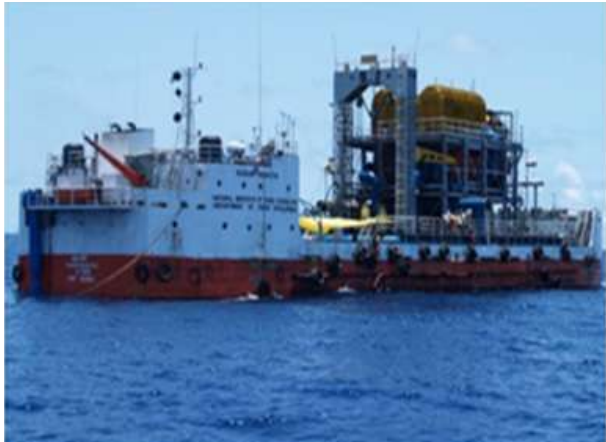
Barge mounted 1 MLD LTTD plant
