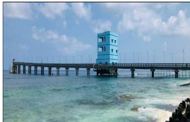
Seawater intake and LTTD plant at Lakshadweep Islands
