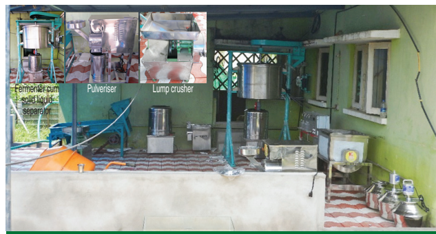
Mechanised organic manure production plant
