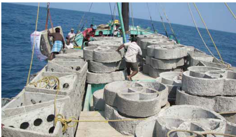
Transporting and deploying reef modules
