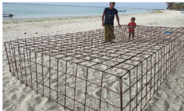
Fabrication of cage for seagrass restoration
