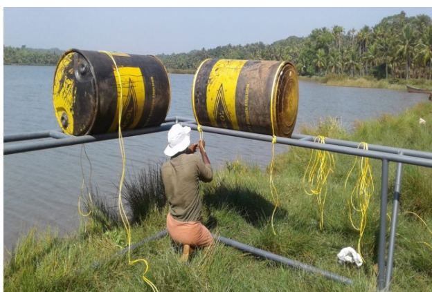
Attaching floats to cage frame by beneficiary
