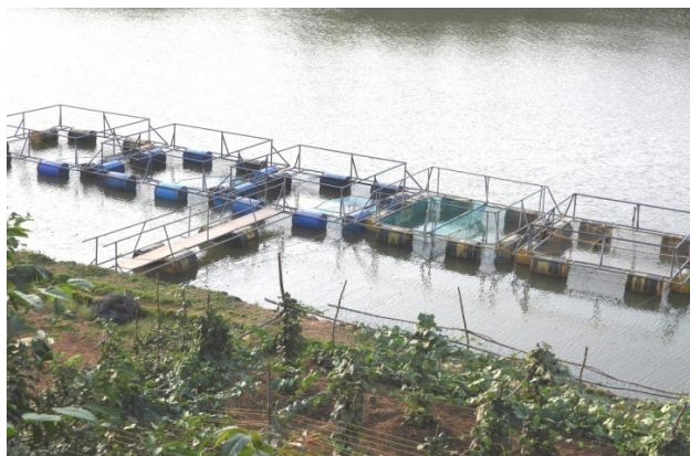
Fabrication of GI catwalk
