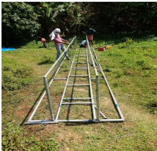
Galvanized iron (GI) cages at Bekal
