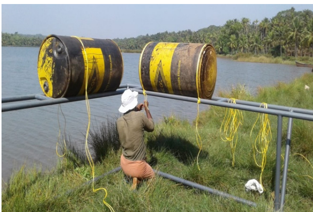
Attaching floats to cage frame by beneficiary
