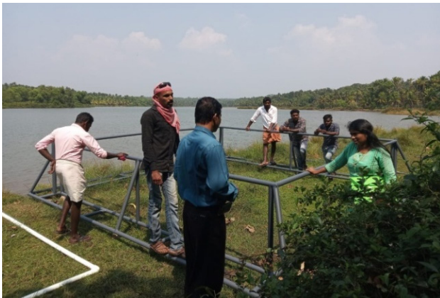
Fabrication of cage frame
