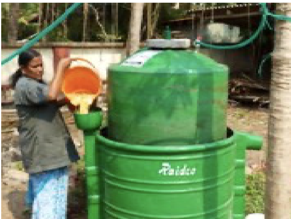
Loading the biogas plant with the bio-waste generated at the canteen and the fish biology laboratory.
