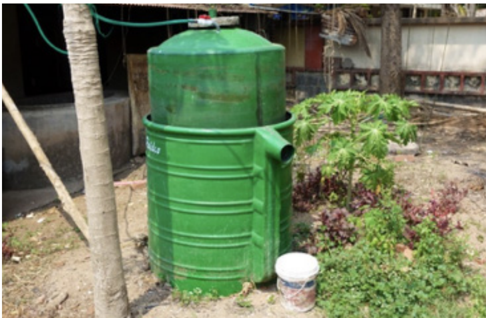
The bio-gas unit at Calicut RS of CMFRI setup with help of The Regional Agro Industrial Development Co-operative of Kerala Ltd. (Raidco). Biogas production from vegetable waste and fish waste was demonstrated in the campus for empowering the public to practice the conversion of waste to wealth
