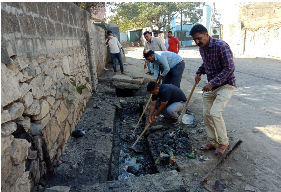
Cleaning of clogged drainage in Veraval
