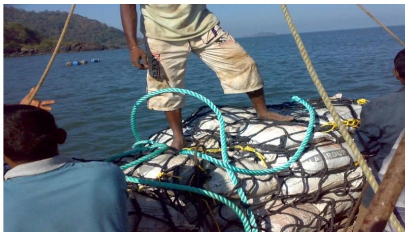
Single point mooring using sand filled bags (Gabbion box)
