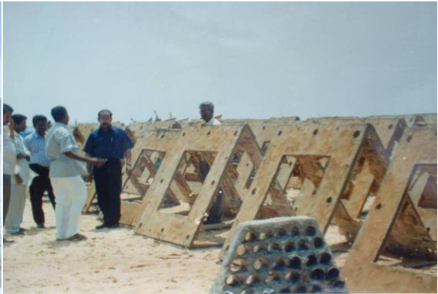
Triangular modules ready for transportation (Poovar, Trivandrum)
