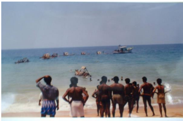
Catamarans with modules being towed to the reef site (Poovar, Trivandrum)
