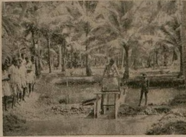
Fixing of velon screen in the sluice gate
