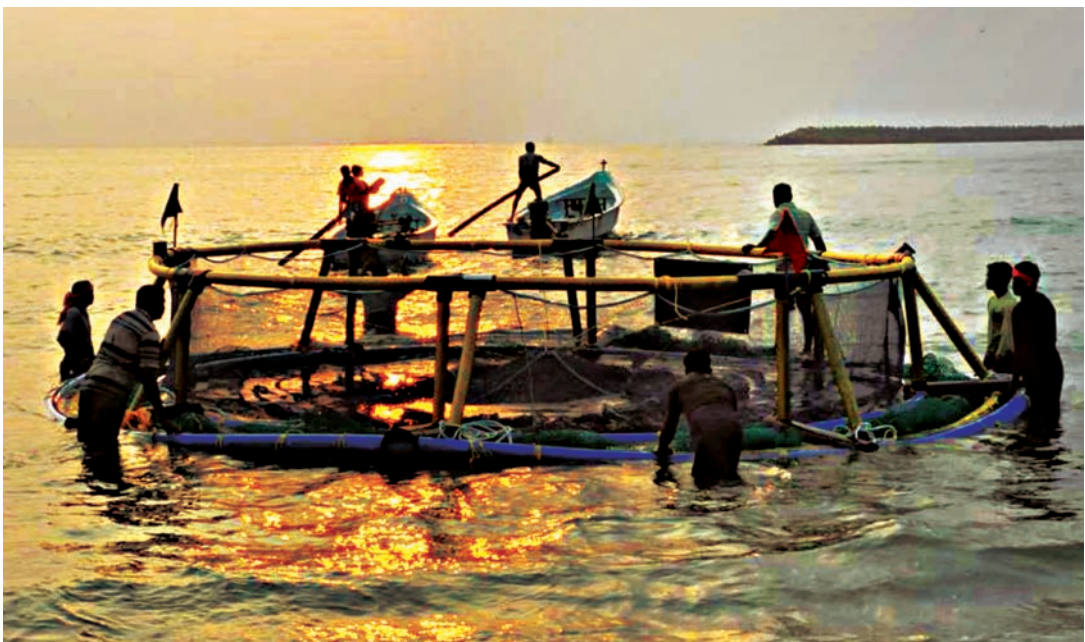
HDPE Cage installation in progress in Kanyakumari coast
