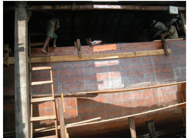
Fig. 2. A multi-day deepsea trawler under construction at the boat building yard, Malpe
