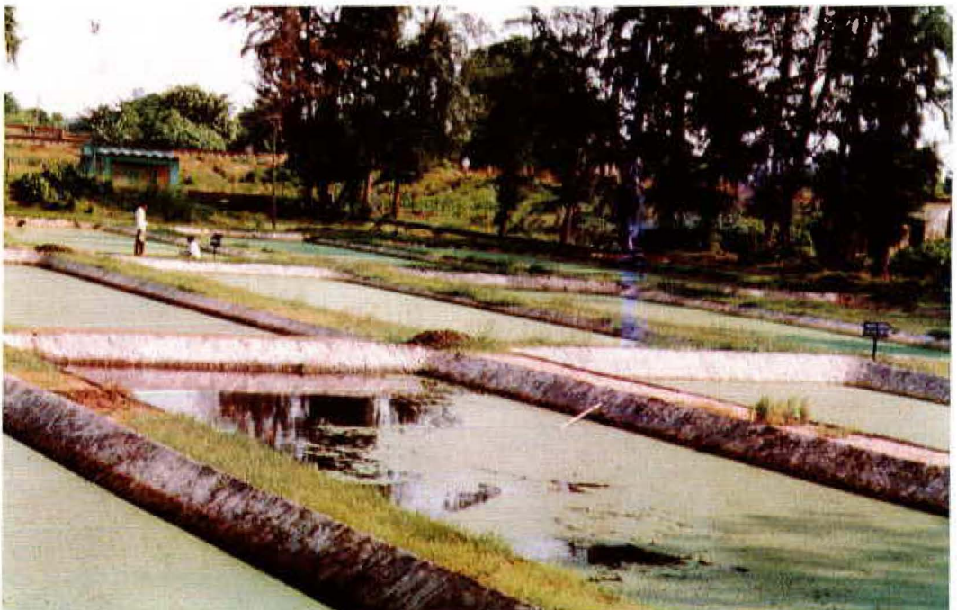
Fig. 3. Treatment of domestic sewage
