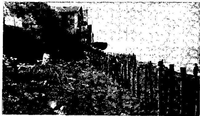
Fig. 4. Another location of severe sea erosion.
