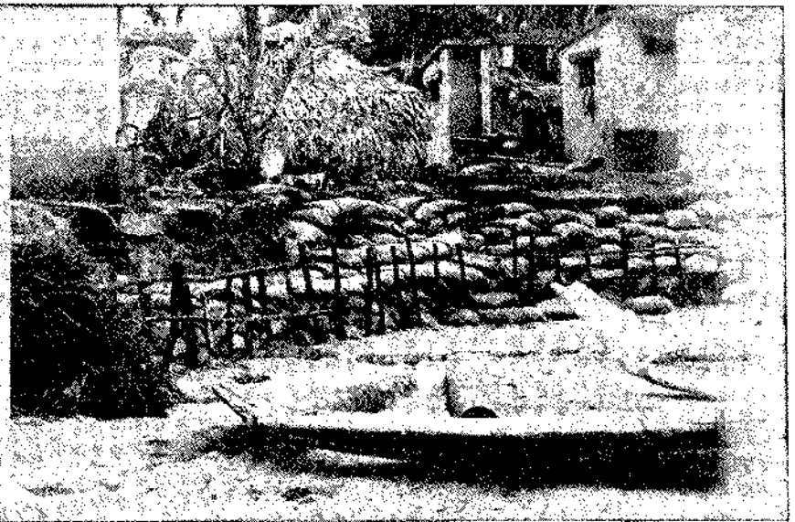
Fig. 5. Sand bags stacked on eroded beach in front of the houses for temporary protection.
