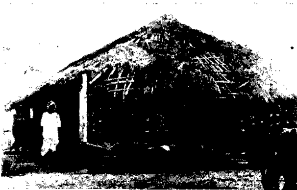
Fig. 4. House in which 200 lives were saved at Nali in Krishna district in 1977 cyclone.
