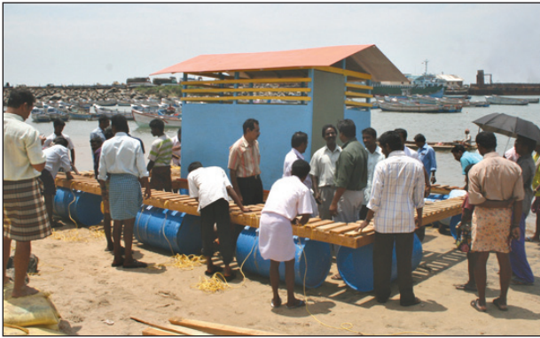
Raft for holding the multiple cages getting ready at Vizhinjam Harbour area
