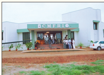
Lab-cum-Office building at South Beach Road, Tuticorin
