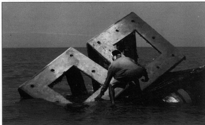
Artificial reef modules being installed at Thikkodi-Moodadi
