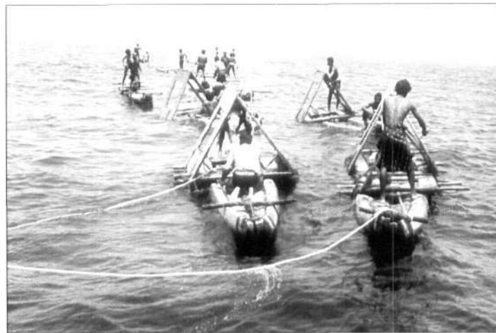
Modules being transported for installation
