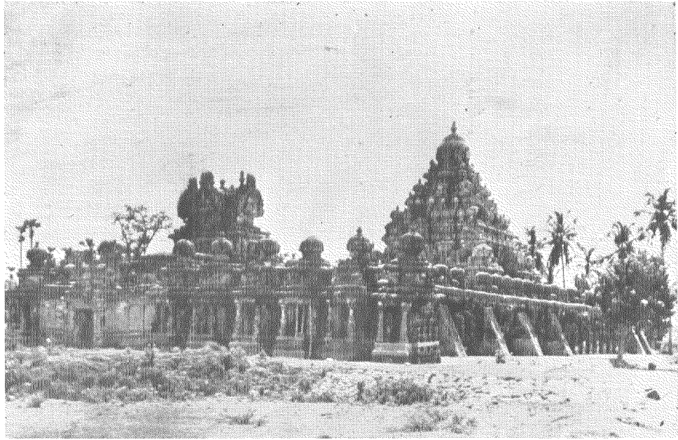
↑ KAILASANATHA TEMPLE AT KANCHI, BUILT BY RAJASIMHA (8th Century A. D.)
