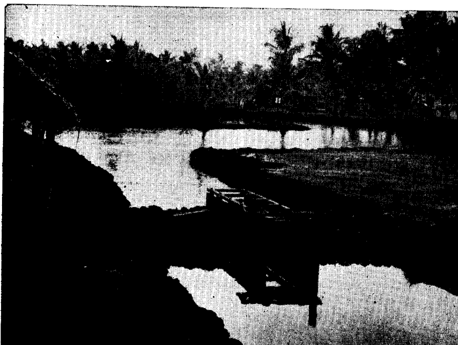
Thoppithati (top frame) to the sluice gate is being fixed.
