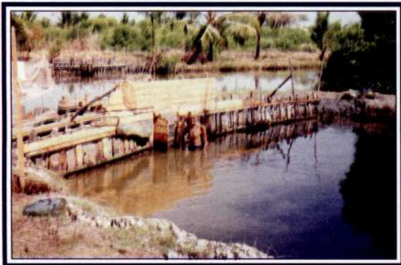
A view of a fabricated sluice
