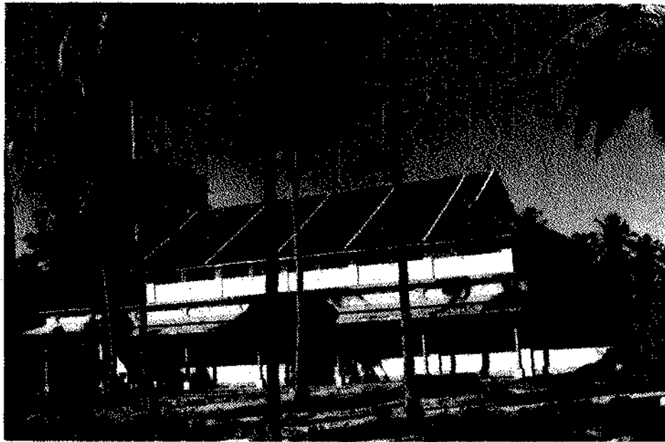
Mariculture complex at Calicut being commissioned
