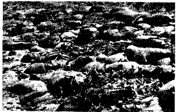
Fig. 5. The sand bags piled up have been shattered by the huge waves at many places at Edavanakkad.
