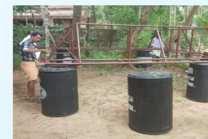
Coating of anti-corrosive paint
