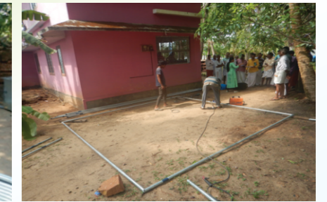
Fabrication of outer cage frame
