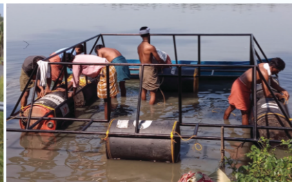
Cage frame attached with floats
