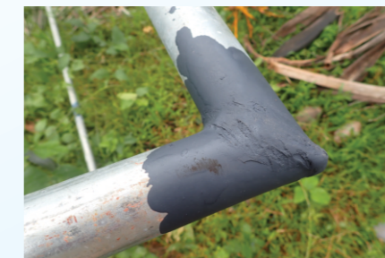
M-seal sealing at the welding joints
