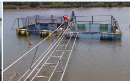
GI cat-walk installation
