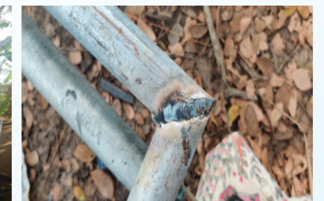
Welding at the corner joints
