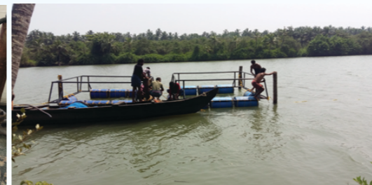
Installing GI cages using bamboo poles
