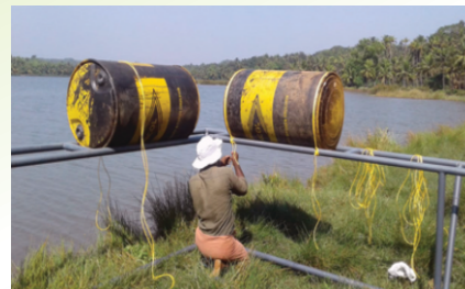
Tying 200 L barrels in GI cage frame
