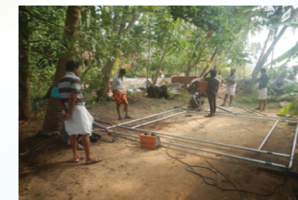
Fabrication of inner cage frame
