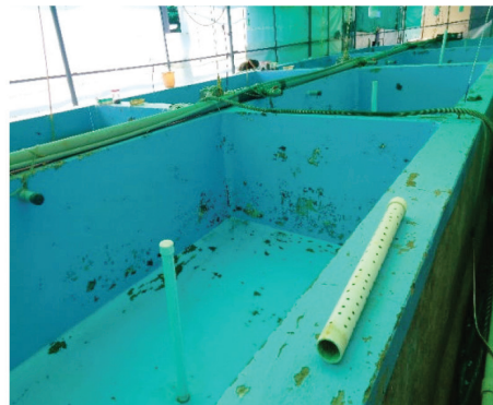
Concrete tanks with central drain
