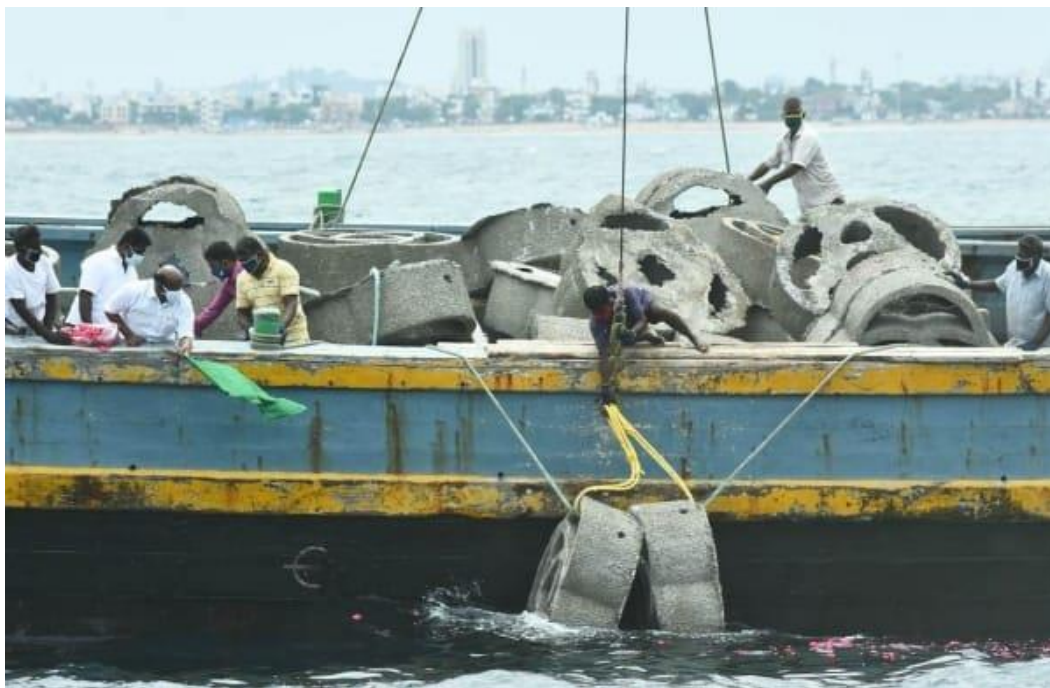
Fig. 35. Flagging off and deploying the reef modules at the fixed coordinates
