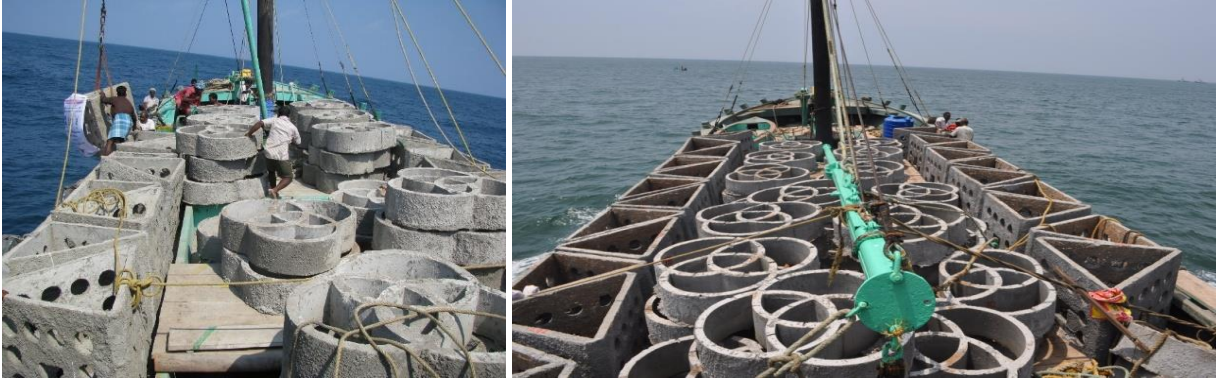
Fig. 36. Deploying the reef modules at the fixed coordinates in different locations
