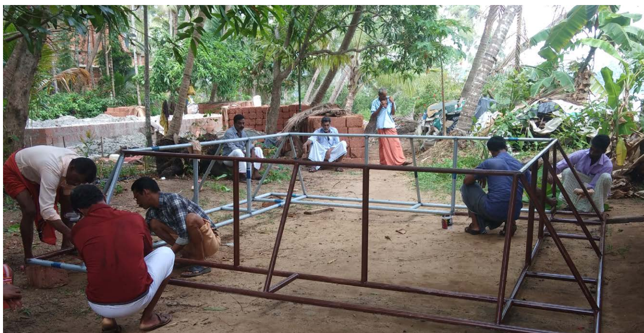
On-field practical demonstration on GI cage fabrication
