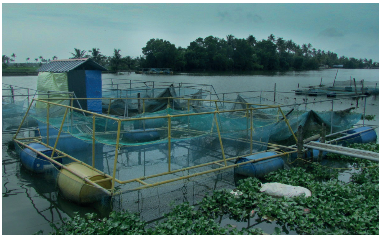
Fig.1 Battery of cage farms damaged
